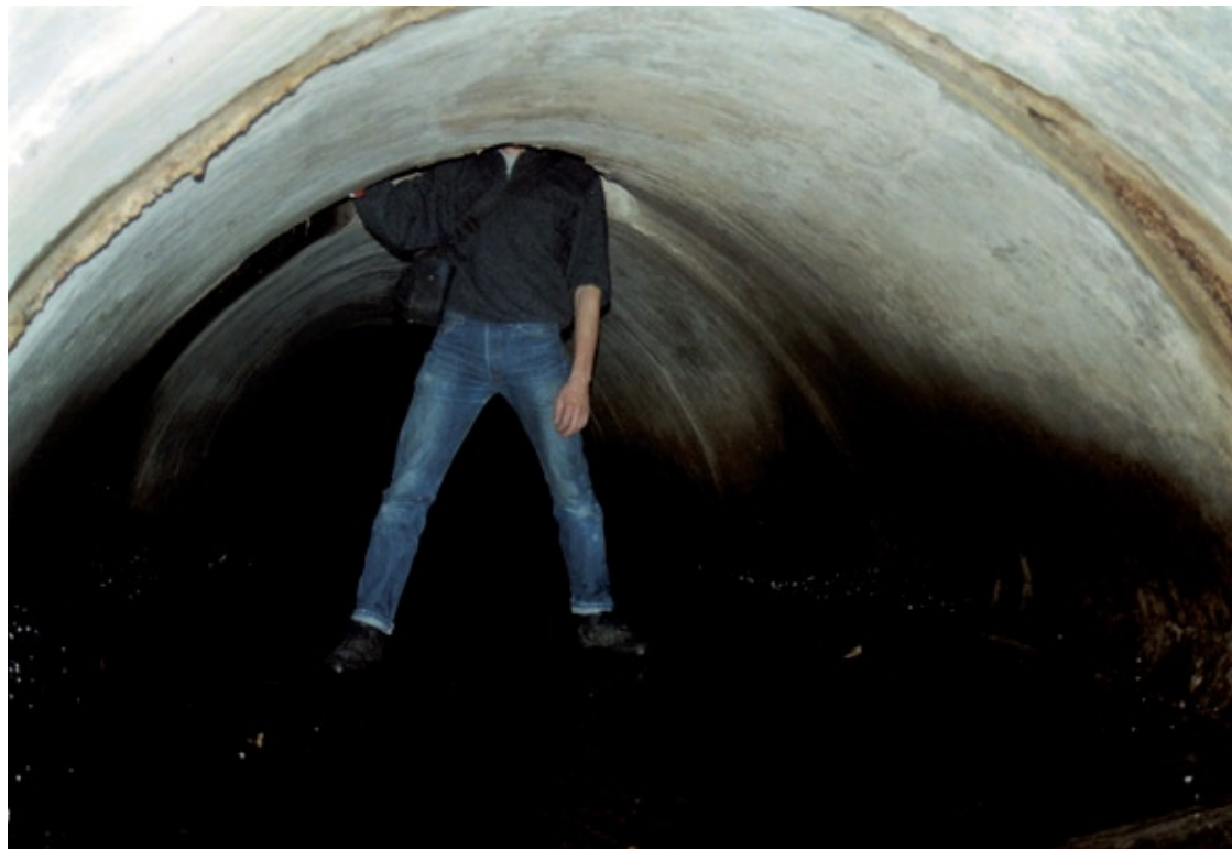
//01.09.06 - The first time in the sewer system. Went with Fiona into an entry shaft, stretched out our backs, and made tags. The largest tunnels of the Berlin sewer system are only about 150 centimetres high. You get a backache really fast. You have to build yourself a vehicle in order to be able to move on further into the tunnels.
